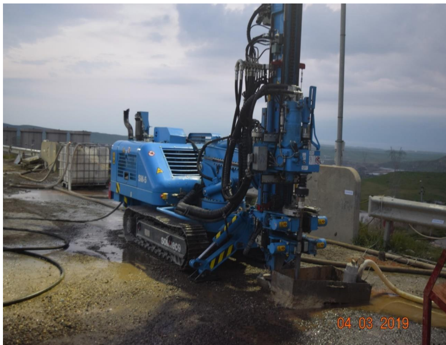
Figure 4: Drilling inside the tunnel and on the body of Mosul earth dam.
